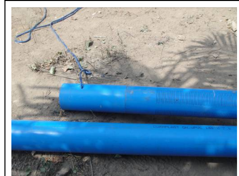
Figure 10. Preparation of the casing for installation
