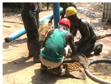
Figure 14. Installation of the clay sanitary seal.
