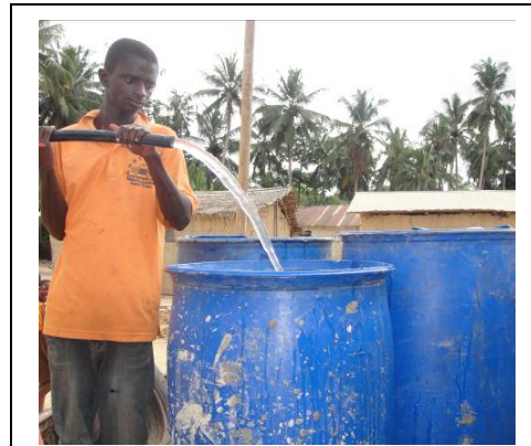
Figure 16. Discharge during development 35 litres/minute
