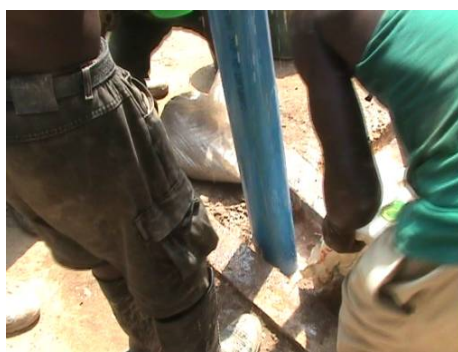
Figure 13. Installation of the gravel pack
