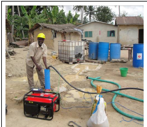
Figure 15. Developing well using a 1HP submersible pump and 2.5 KVA generator
