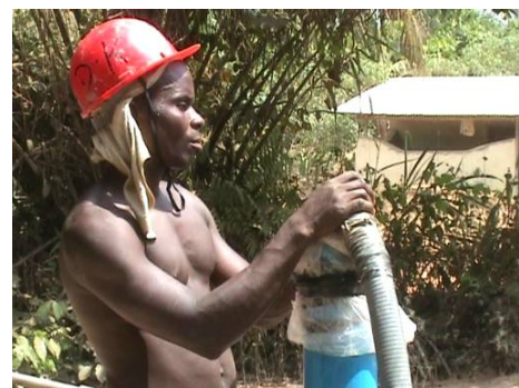
Figure 12. Flushing the drilling polymer out of the well
