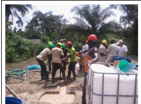
Figure 9. Well drilled using rotary jetting to a depth of 25.5 m
