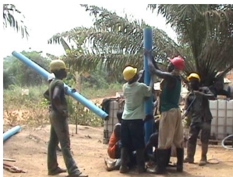
Figure 11. Installation of the casing
